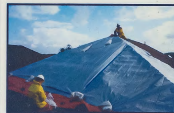
Phil Hurst and Rod Taylor tarping a roof
