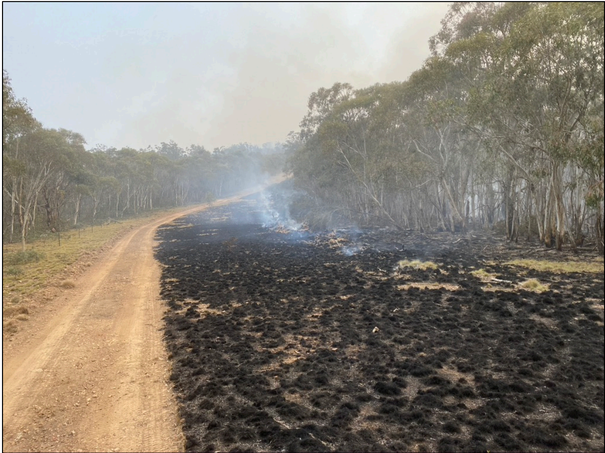
A good example of a boundary fire trail – ideally the cleared country should extend as shown but on both sides of the boundary fence.
